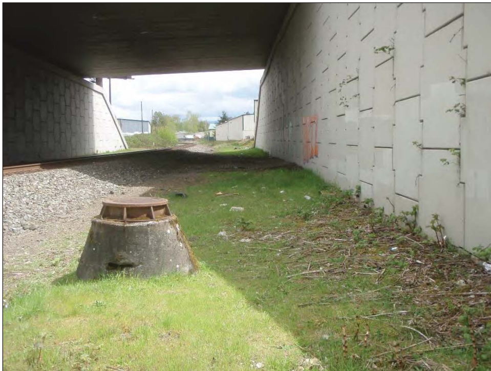
Photo F. View east of storm manhole and lack of railroad ditch (does not daylight to east). Photo date April 20, 2017.
