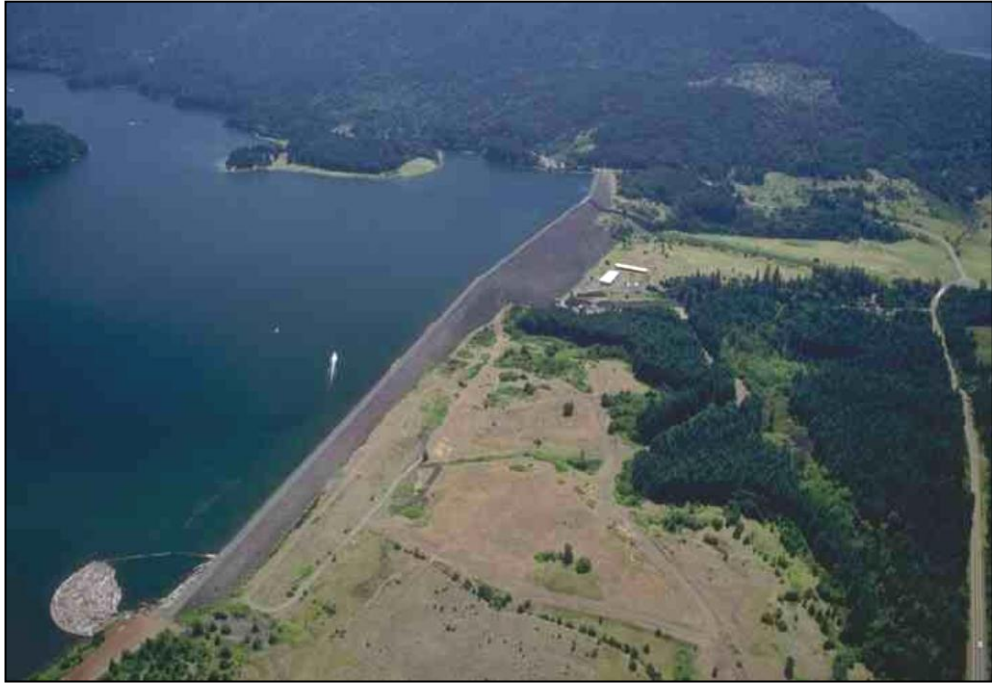
Figure 2. Fall Creek Dam and Reservoir in Lane County, Oregon
