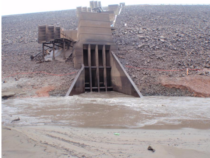
Figure 3: Fish Horns (upper left) and one of the two regulating outlets (lower center) at Fall Creek Dam, Lane County, Oregon. View looking downstream during a drawdown as reservoir water enters the regulating outlet.
