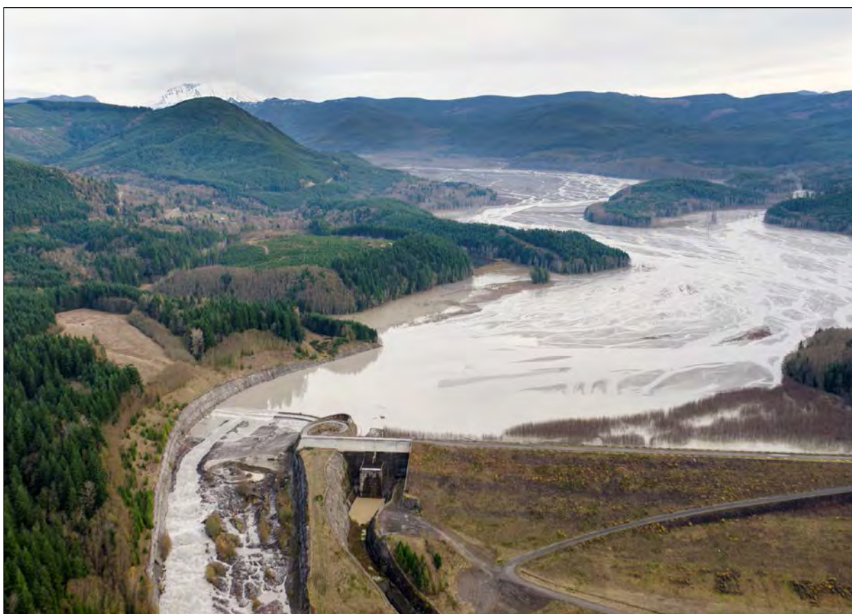
Sediment retention structure and upstream sediment plain on the North Fork Toutle River.
