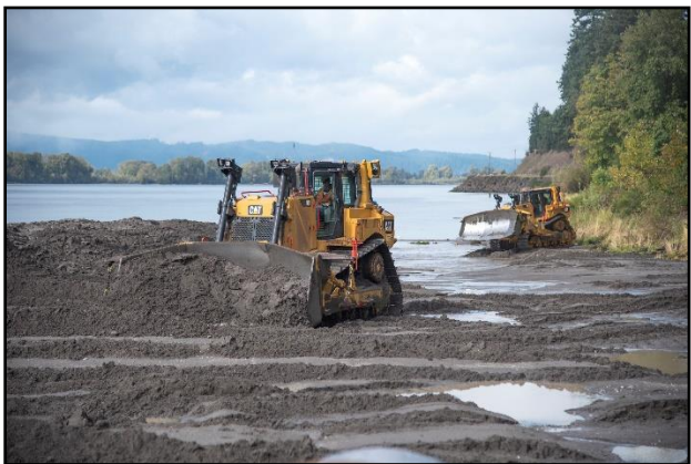
Bulldozers move the sediment into place after it exits the pipeline.
